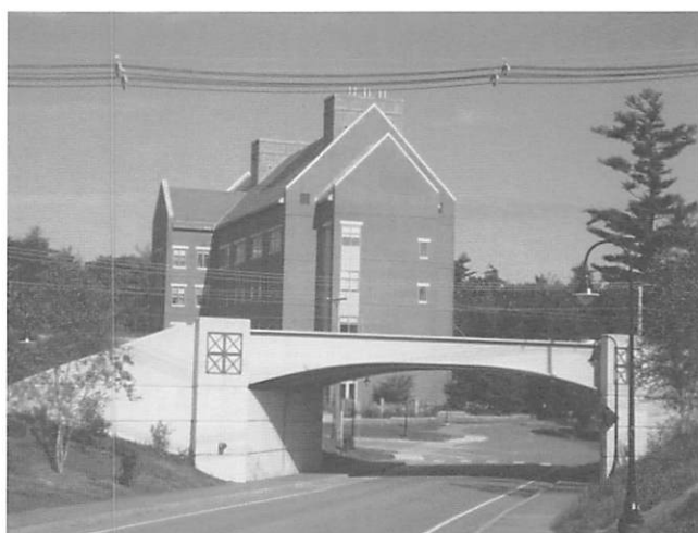
図-5 UNH (Material Recycle Center)
