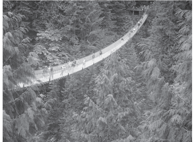
写真-10 Capilano suspension bridge
