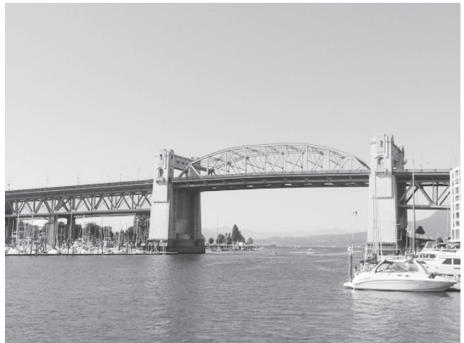
写真-6 Burrard street bridge
